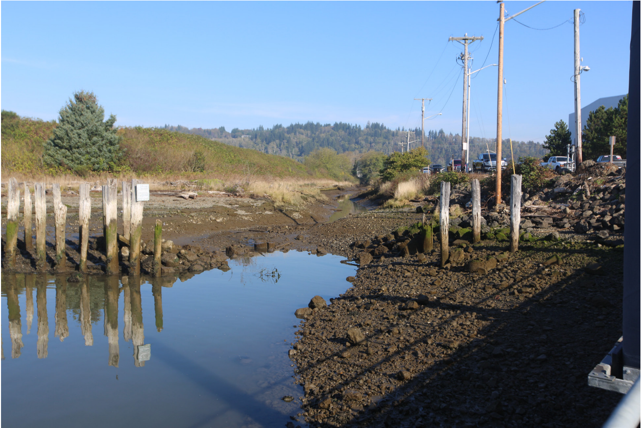
Photograph 1 Offsite Ditch West of Port. Photograph Taken Facing North from Public Boat Launch, 10/14/2022.
