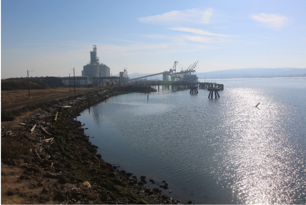
Photograph taken facing east approximately 150 feet east of Fry Creek outlet on October 14, 2022. Terminal 2 and shiploader are visible in the background.
